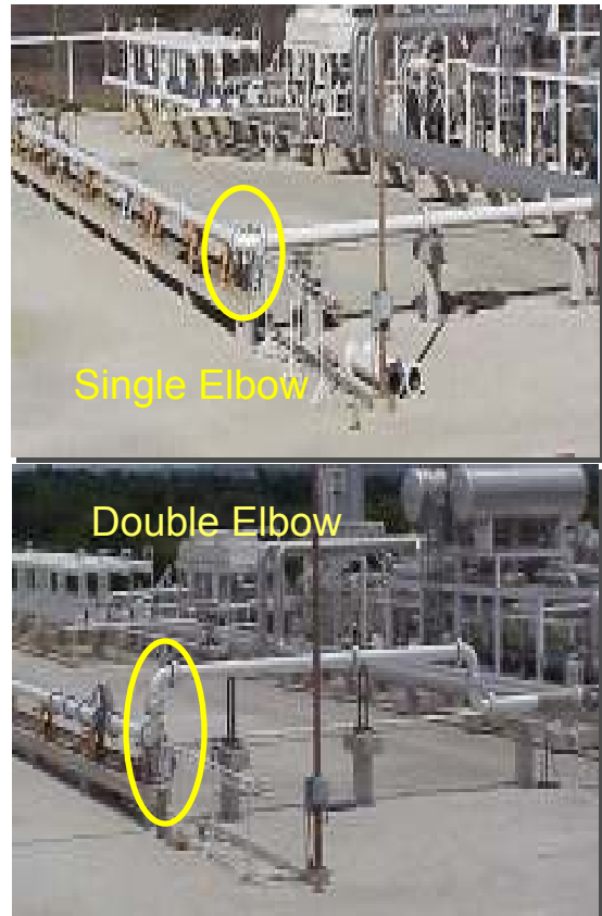
Figure 3. Two common upstream piping configurations.
